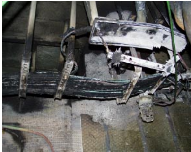
FIGURE 5 Fire damage to deckhead cables and fittings
