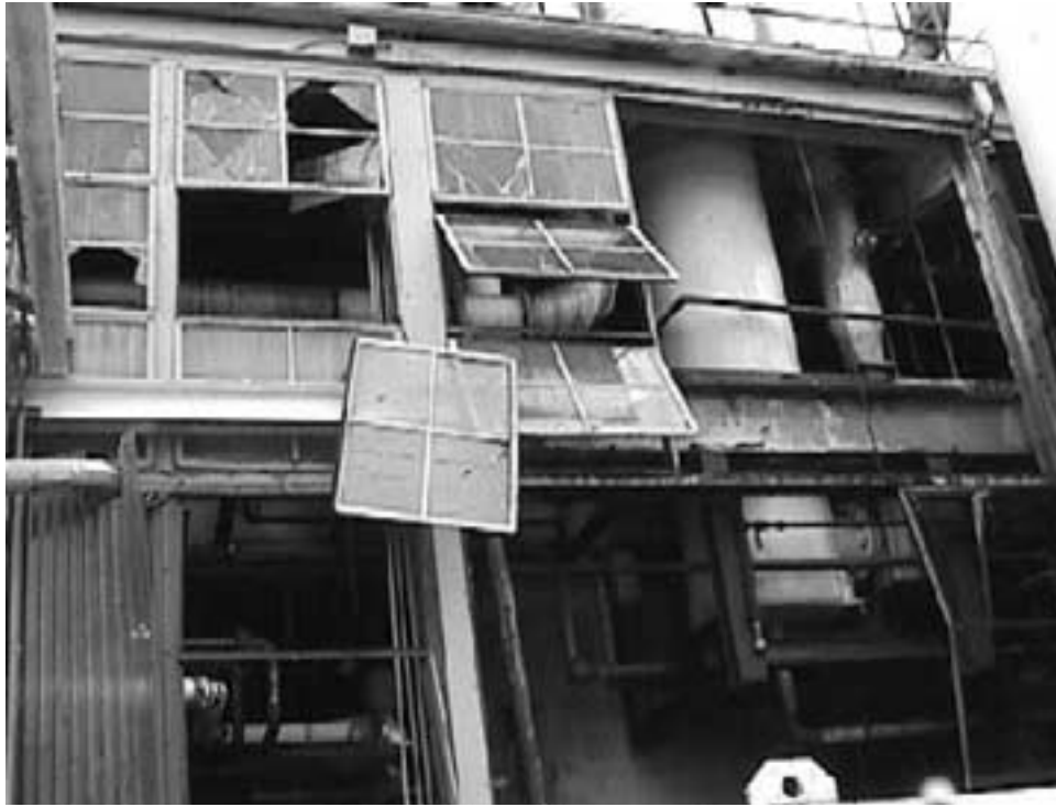
Figure 13: Building 11's Blowout Panels and Window Frames
