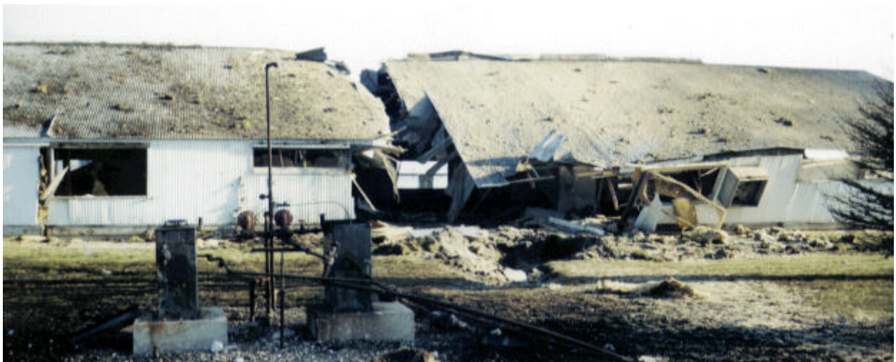
Figure 12. Damage to Turkey Barn (1g) Caused by Impact of Large Tank Fragment
