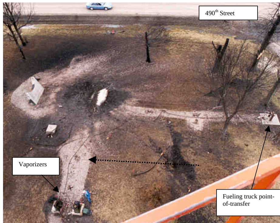
Figure 7. Aerial View of Tank Area
