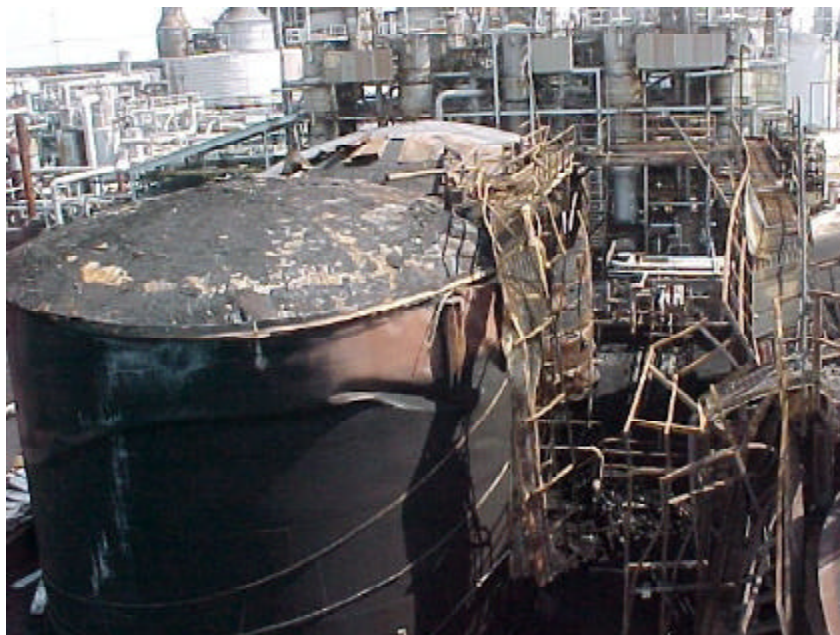
Figure 3. Tank 394 in foreground and remains of catwalk, from the north.
