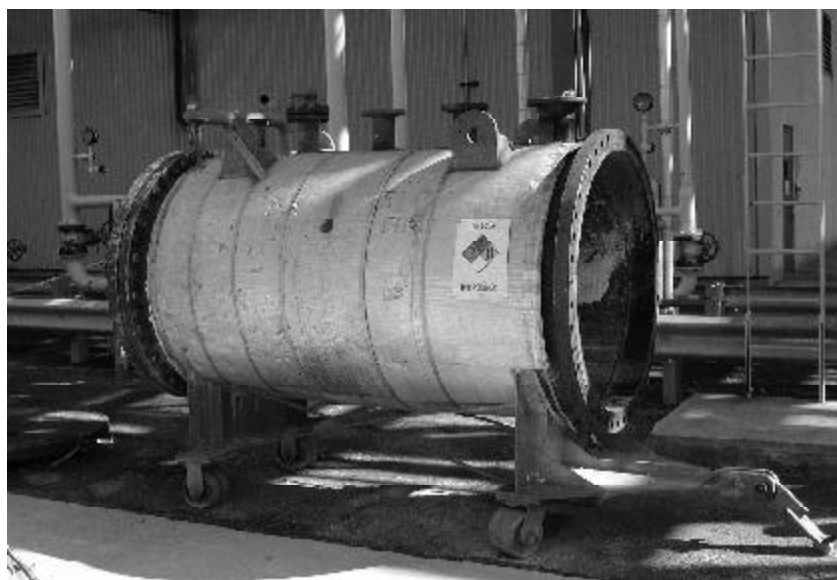
Figure 3. KD-502 polymer catch tank (actual vessel with one cover removed).
