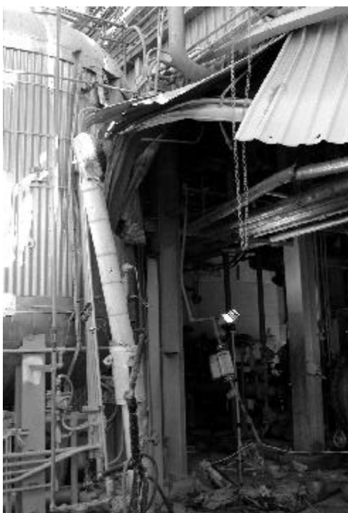
Figure 5. Damaged girder.
