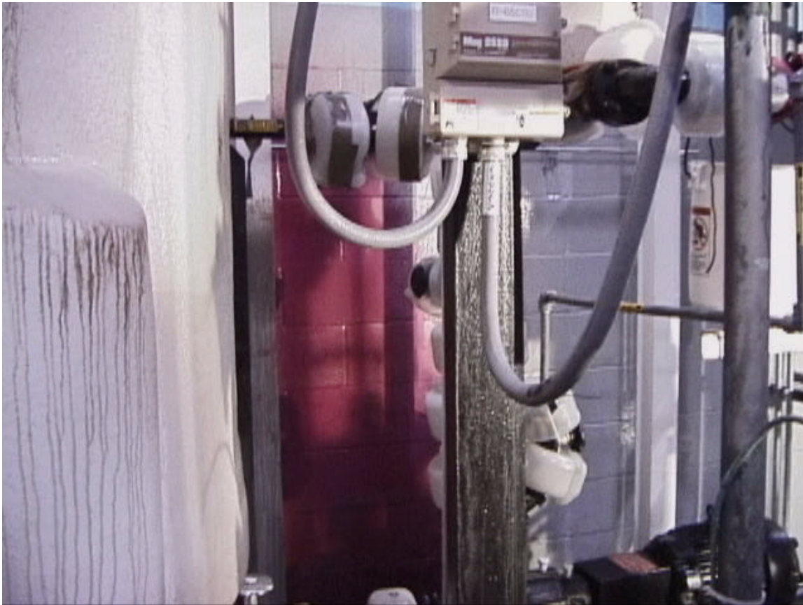
Chemical berm area. Pump located behind unistrut support in center of picture. Notice spray pattern on wall.
