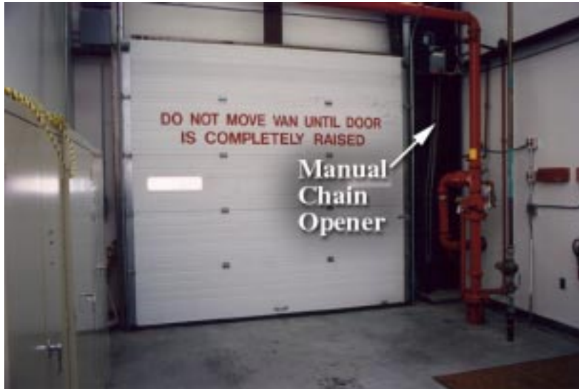
Exhibit 2-6. Emergency Control Center Door
