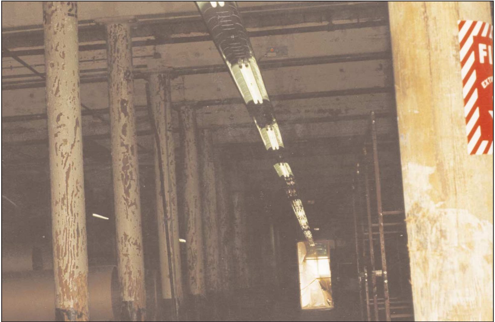
9. Typical mill building construction with heavy wood beams and thick wood floors.
